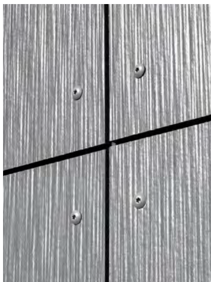
Hardie® Panel Screw Fixing
